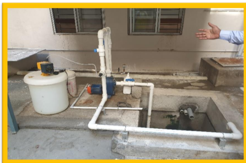
Disinfection system with a treatment capacity of 500Litres/Day Located in the hospital block
