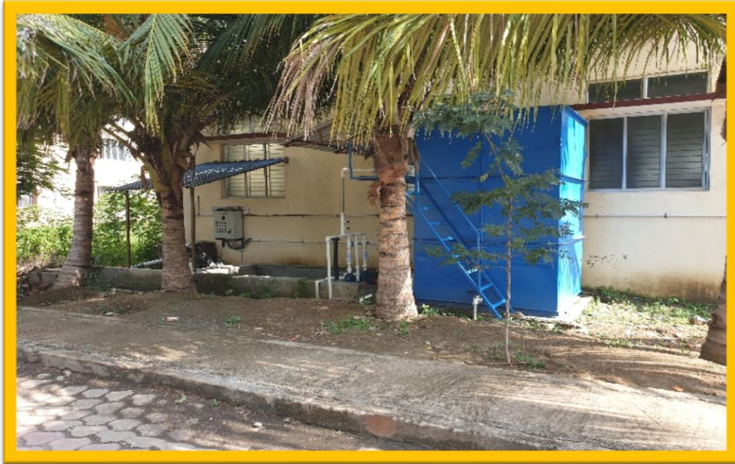
Central collection area for Biomedical Waste
