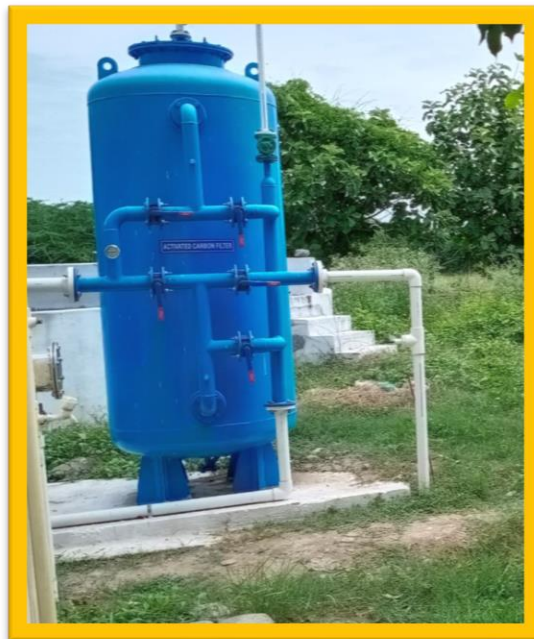
Activated Carbon Filte Pressure Sand Filter
