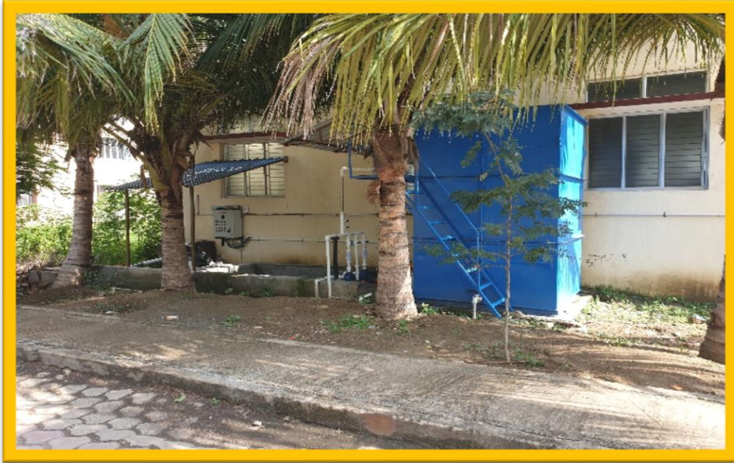
Central collection area for Biomedical Waste
