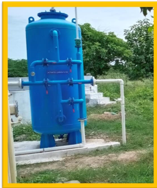
Activated Carbon Filter Pressure Sand Filter
